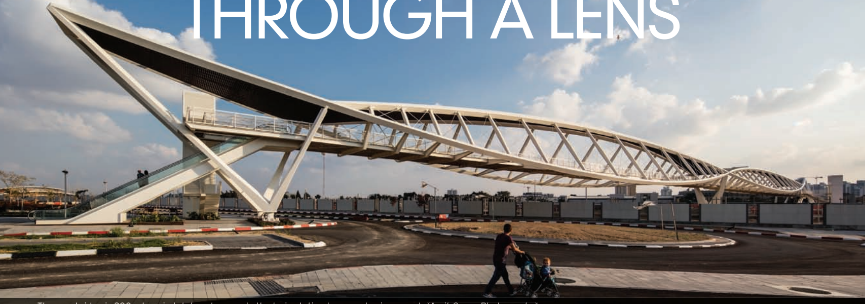
The new bridge is 200m long in total, and connects the train station to a new business park (Amit Geron Photography)
