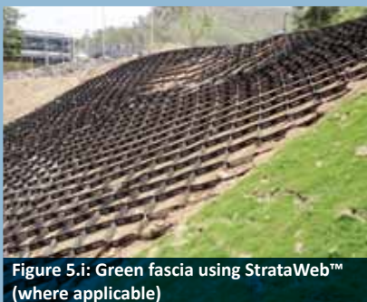
Figure 3: Laying of StrataWeb™
