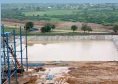
Reservoir lining, Gandhidham
