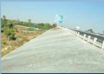
ROB – NH 202, Andhra Pradesh
