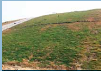
Landfill lining, Delhi
