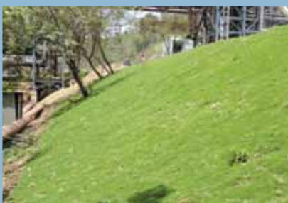
Slope protection for gas plant
