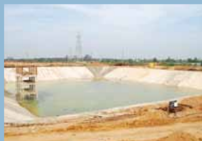
Reservoir lining, Chennai
