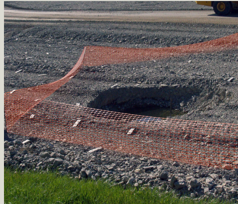
Subsidence found at the base of the embankment
